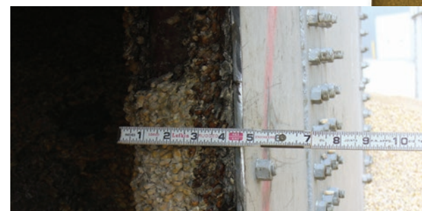
Kernels of corn often get stuck to the walls of the bin, obstructing the flow of the corn.
